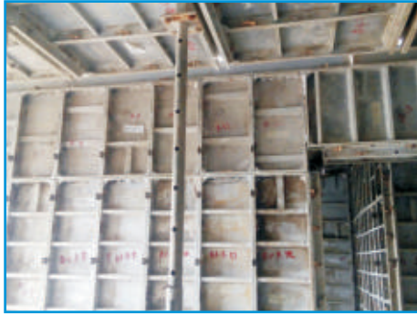
Aluminum Shuttering For Rcc Wall Structure
