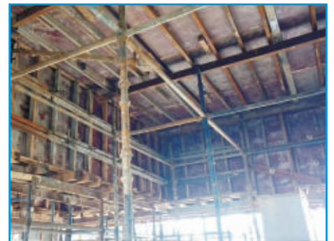
Cuplock Shuttering For Girder Slab
