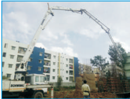
Concreting With Boom Pump
