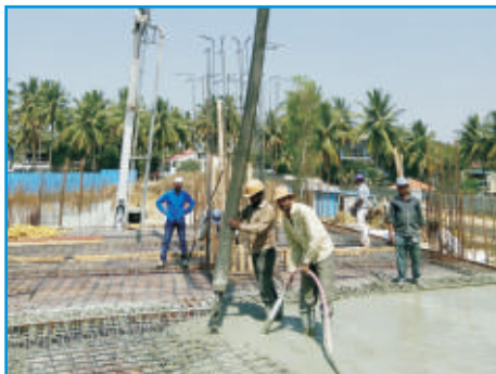
Concreting With Boom Pump
