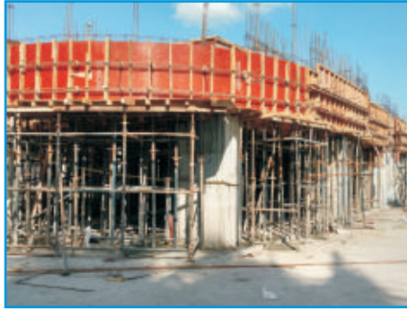
Plywood Shuttering For Curved Balcony
