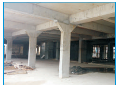
RCC Slab For Podium Parking
