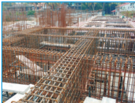
Girder Slab Reinforcement
